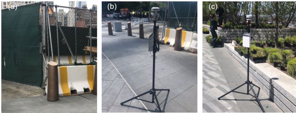
Figure 3. Small scale feature that may obstruct the wind on site: (a, b) construction elements, (c) landscaping.
